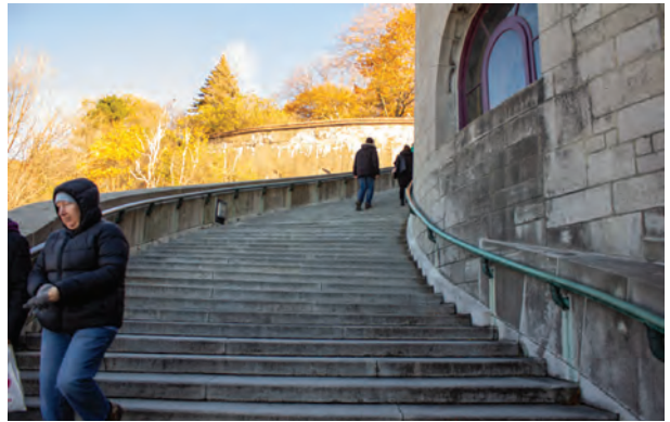
Stairs leading up to the top of the Oratory
